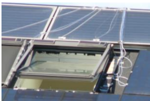
Figure 4. Pressure taps location on site (17.1° open)
